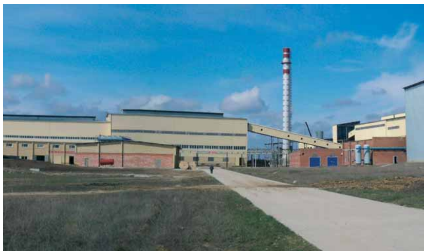
▲ YugRosProdukt, a specialised container glass producer in Russia, constructed a float line in the south of Russia, which began production at the end of 2009.
