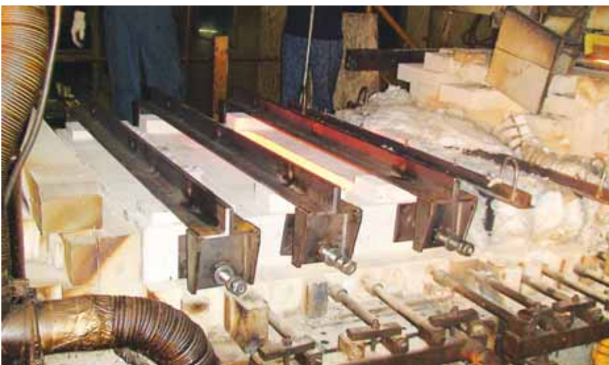
▲ Hot replacement of equalising section roof.
