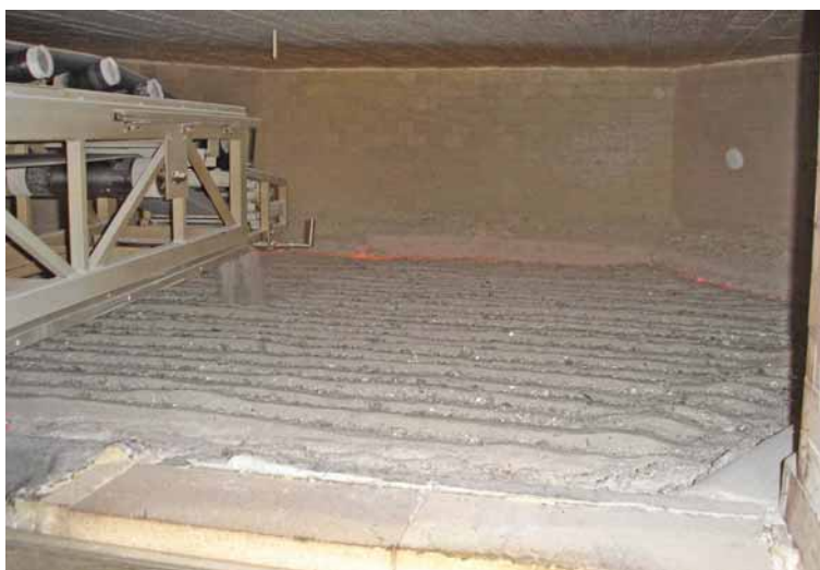
▲ A typical batch blanket in an Electroglass all-electric melting furnace.
